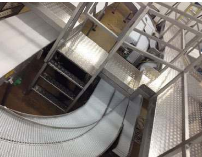
Conveyors and walkways in packing hall of pie manufacturer
